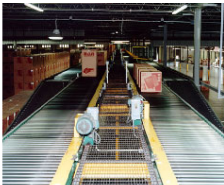
Ceiling supported conveyors "A" transporting loads from production to warehousing.
